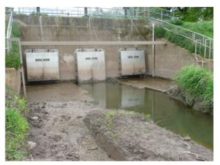
Fig 1:Typical flood defence doors/flaps.
